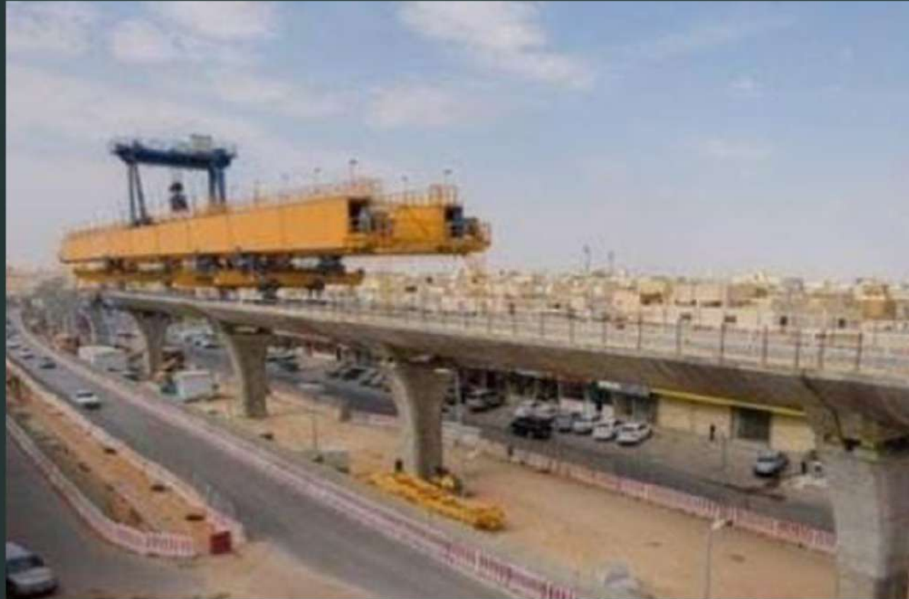
RIYADH METRO –SYSTEM UNDER CONSTRUCTION
