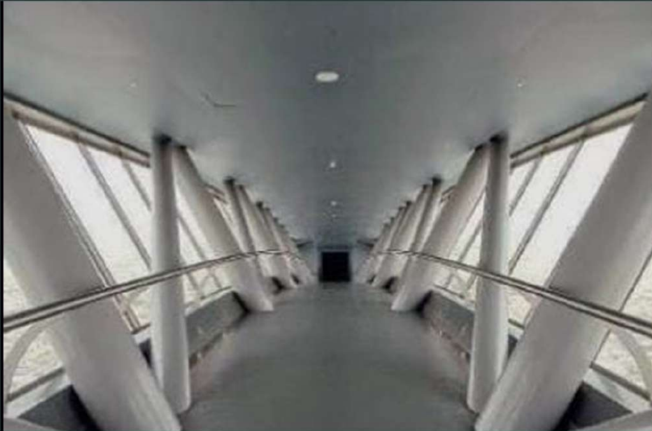
SKYBRIDGE – KINGDOM CENTER
