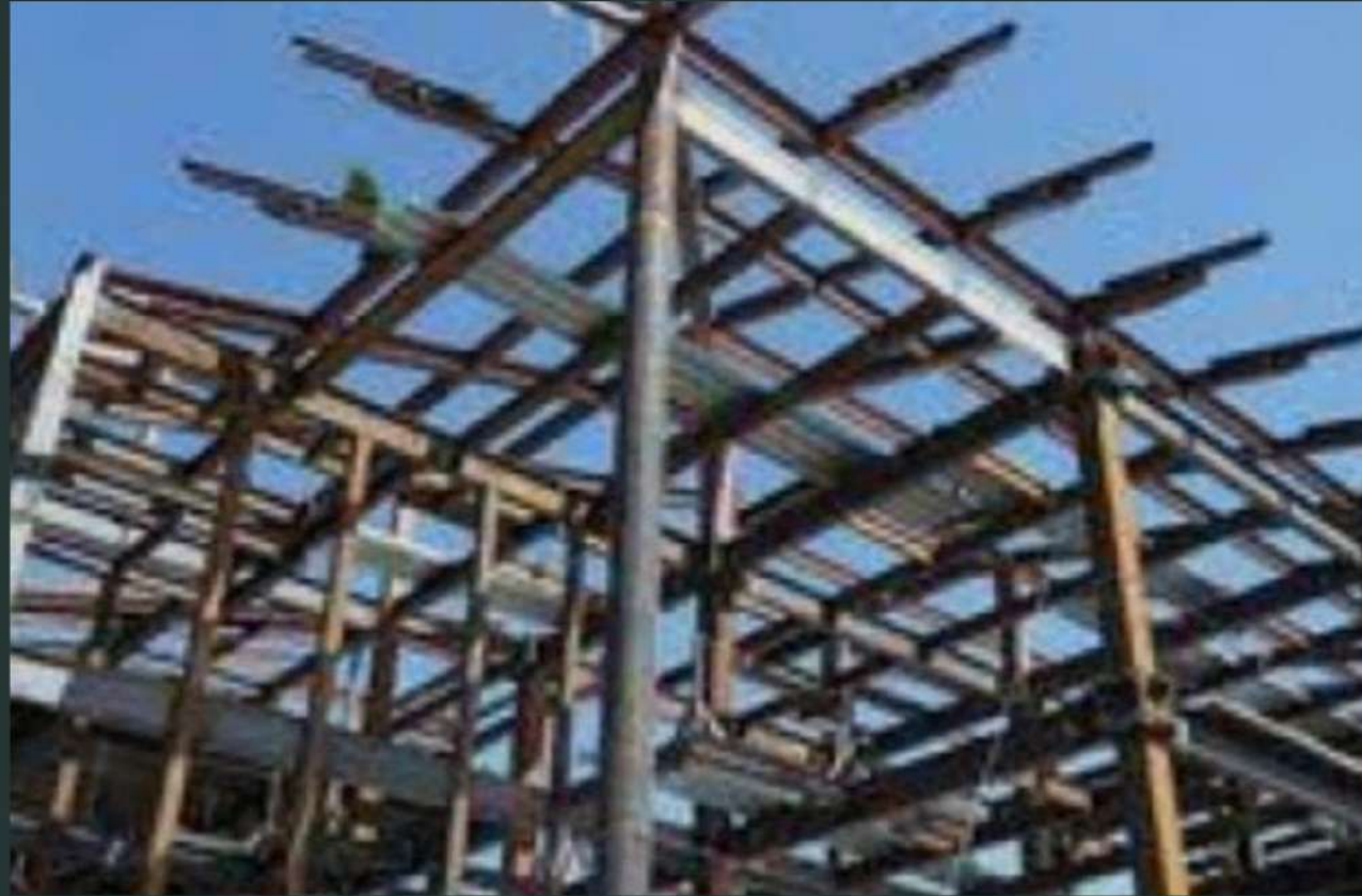
STEEL FRAME STRUCTURE
